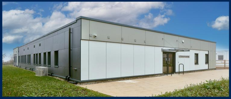
Central installed an EQUITONE UK Rainscreen Cladding System creating a dark grey uniform aesthetic. This was a high-performance, Premium, fibre cement panel. Giving the full creative scope of modern cladding systems with the performance levels required for contemporary buildings.
